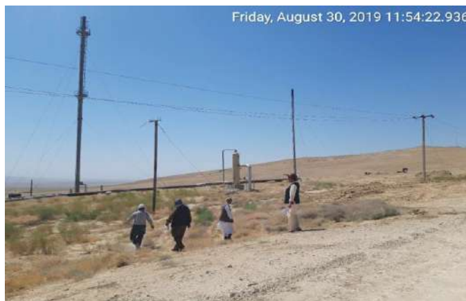
Air pollution prevention system (H 2 S combustion)
