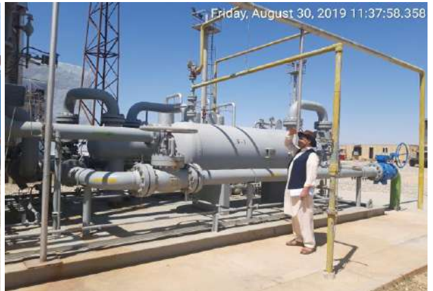
Amine Plant (Sulfur separation)
