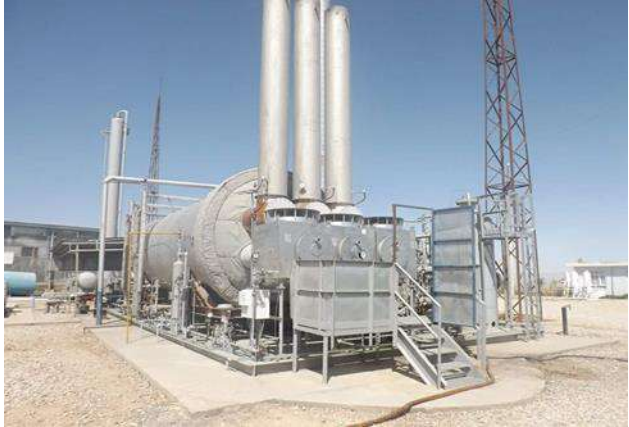
Amine Plant (Sulfur separation)
