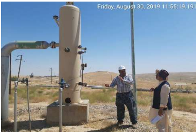
Air pollution prevention system
