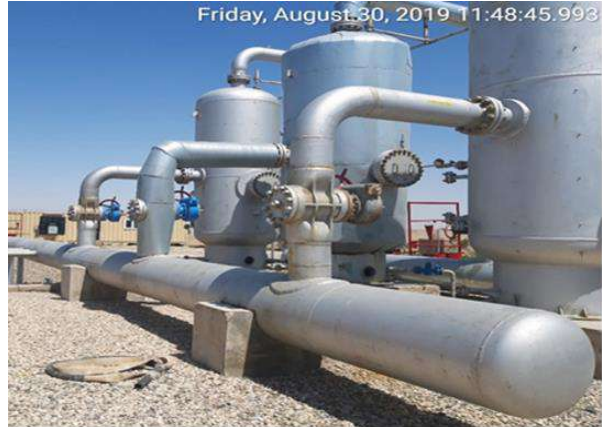
Amine Plant (Gas purification system)
