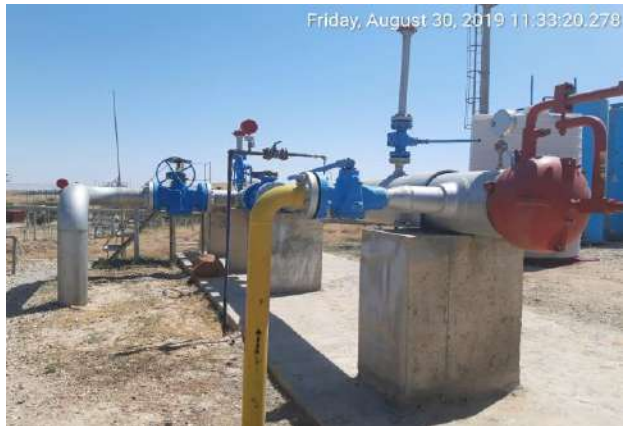
Amine Plant machinery
