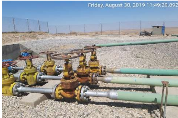
Amine plant (Gas inter to the system)
