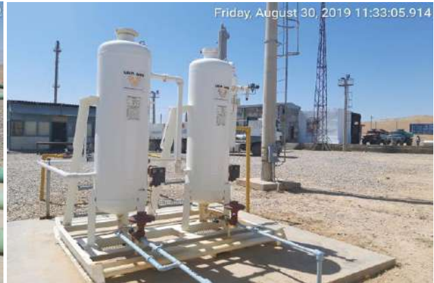
Amine Plant machinery
